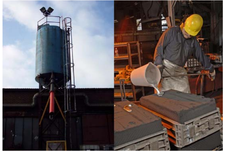
Above: Waste sand silo with new collection pipes at the foundry
